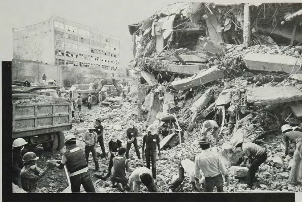
▲ A series of earthquakes devastated Mexico City in September. One of the quakes registered 8.1 on the Richter scale. The entire metropolitan area was affected.
