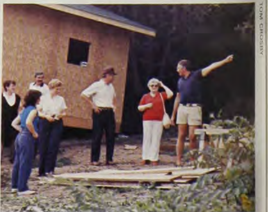
▲ (Middle) Construction on the friary proceeded quickly. After the foundation was in place, carpenters like Joe Antonoli worked on the original framing.
